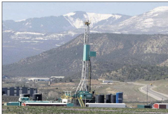
A natural gas well pad sits in front of the Roan Plateau near the Colorado mountain community of Rifle, Colo. Significant amounts of natural gas on federal lands are being wasted, costing taxpayers tens of millions of dollars each year and adding to harmful greenhouse gas emissions, a congressional investigation has found.
