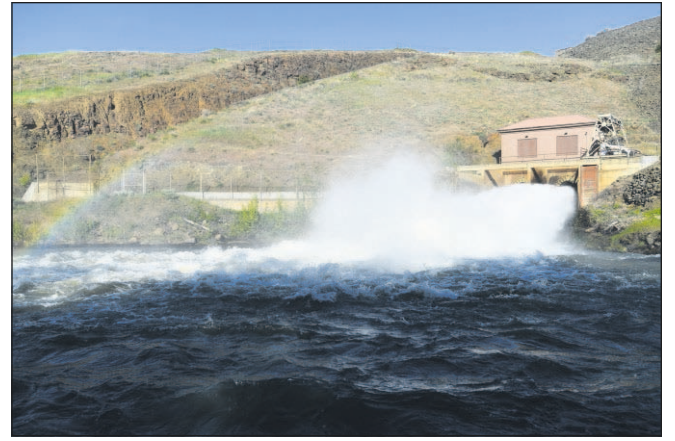
Staff photo by E.J. Harris Water streams out of the McKay Reservoir on Monday and into McKay Creek outside Pendleton. Water is being released from the reservoir to help fish runs in the Umatilla River, which is already running at low summer levels.
