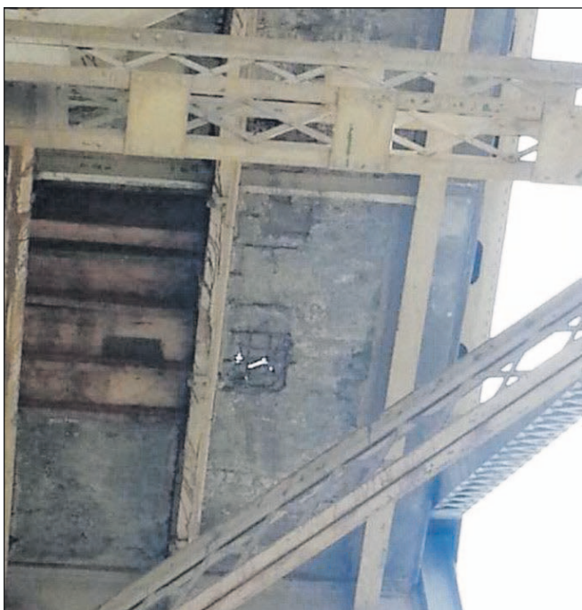
Photo contributed by Washington Department of Transportation A one foot wide hole in the deck of the bridge from Washington to Umatilla, shown from the underside of the bridge, is being repaired.
