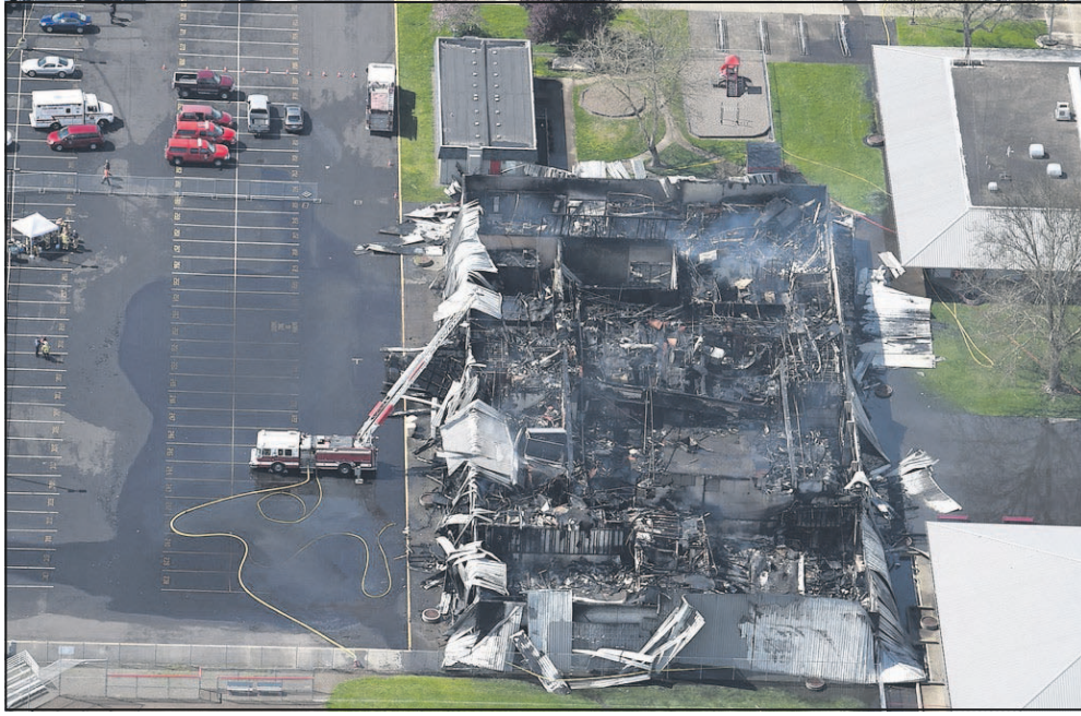
A lone Albany Fire Department ladder crew stands vigil over the smoldering remains of South Albany high school's cafeteria on Wednesday in Albany.
