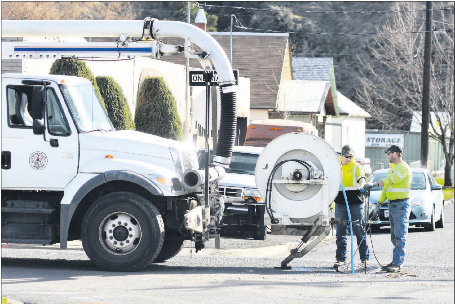
A city of Pendleton work crew cleans a sewer line in February at the corner of Southwest Emigrant and 16th Street in Pendleton.
