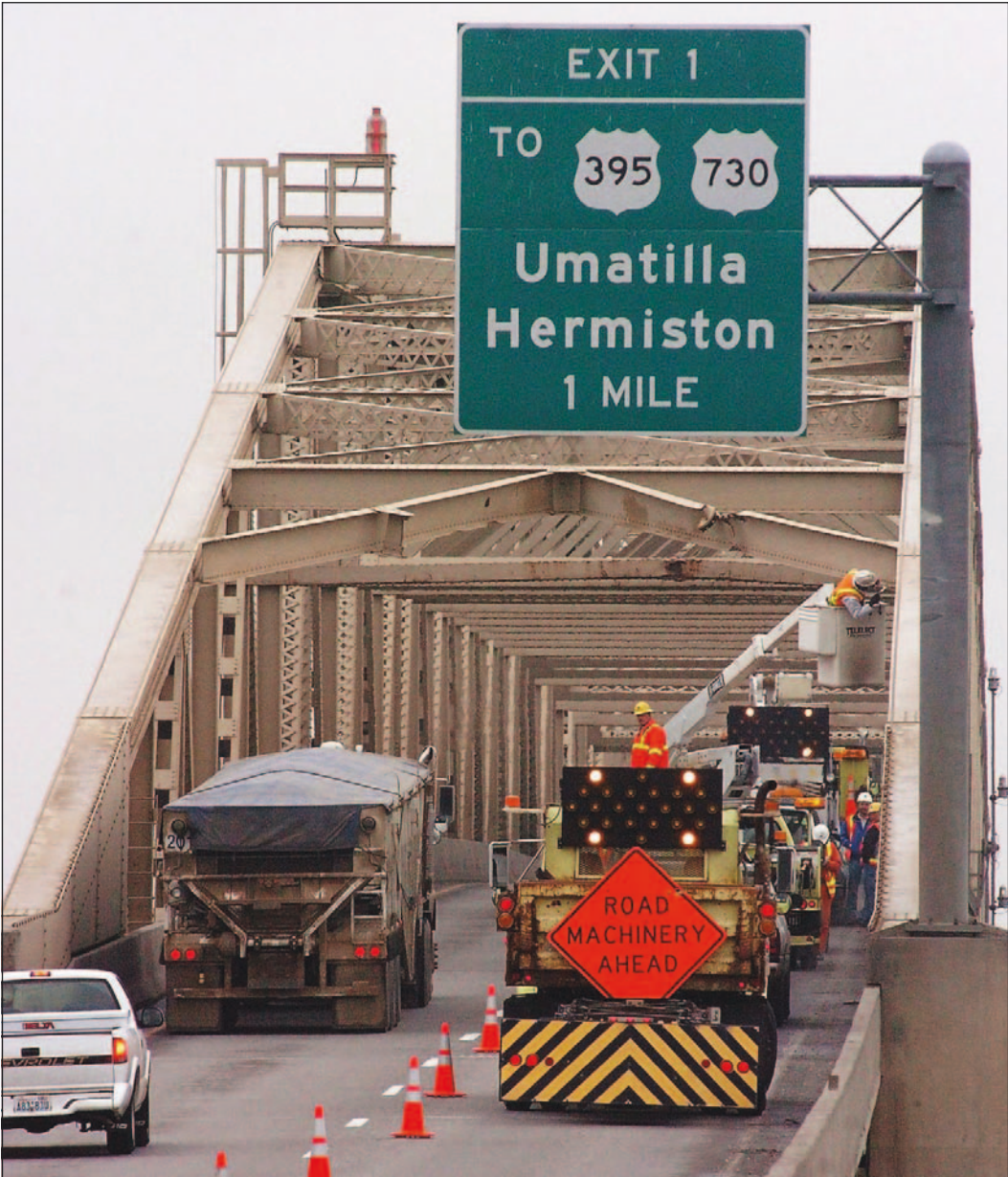
A work crew from the Washington State Department of Transportation Bridge Preservation Office inspects the steel cross beam on the southbound Interstate 82 bridge spanning the Columbia River. The bridge was damaged in 2008 when a oversized semi-truck carrying a log loader crane hit the beam.
