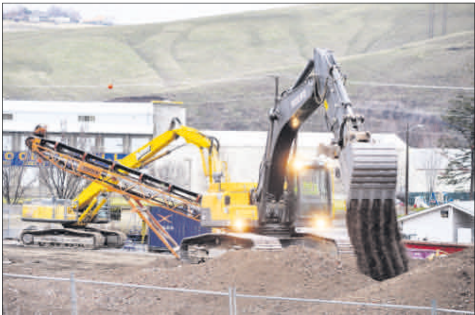
An excavator is used to move dirt at the old St. Anthony Hospital demolition site Wednesday as the project nears completion in Pendleton.
