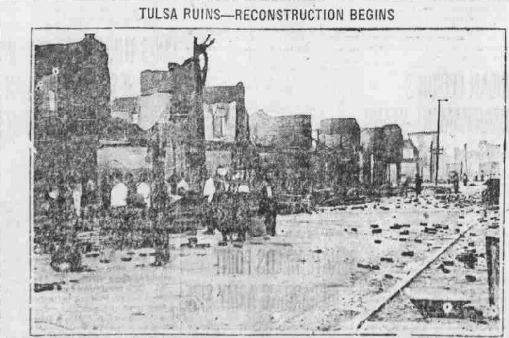
Oklahoma has begun rebuilding the negro section of Tulsa, where many homes were burned down by race rioters and the inhabitants left homeless. This picture shows the extent of the ruin—like a scene in the devastated area in France.
