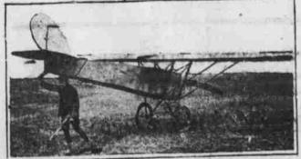
Claim to the world's smallest flying airplane is made by the Rieselet brothers of Johannisihal, near Berlin This plane, shown shows, weights 352 pounds, is 22 feet wide from tip to tip, can attain a speed of 66 miles an hour, and consumes only six gallons of gasoline an hour, a low record for airplanes.
