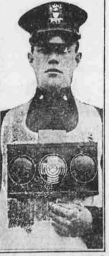
New York police will soon b walking traffic towers, when this new signal device is put in general use. It's a three-way electric lan tern which hangs around the officer's neck. The lights are red, yellow and green. A reflector above illu-minates the officer's face.
