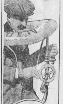
A Paris inventor has turned out a life preserver that has a rudder, propeller and a sail. A hand crank runs the propeller.
