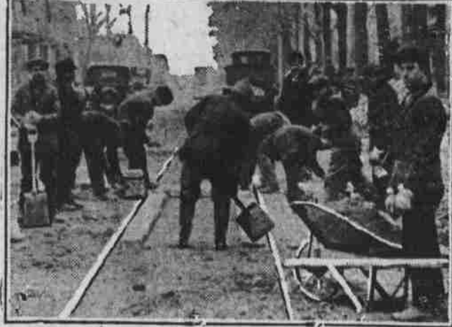
Detroit is out for a finish fight to get better and cheaper street car service. Workmen are shown here laying tracks for the new city-owned line in St. Jean street, despite efforts of the private company to prevent it.
