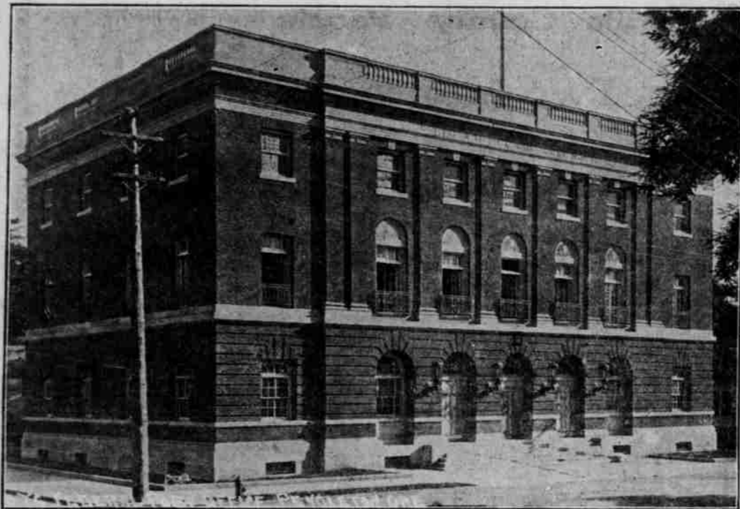
Pendleton Federal Building
