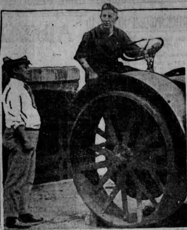
ELGIN, ILL.—When a strike of traction employees deprived Elgin of electricity, motor vehicles filled the gap for small power users. Editor Harry T. Saylor is watching the Elgin Daily Courier. The tractor is coupled to a large dynamo in press room.
