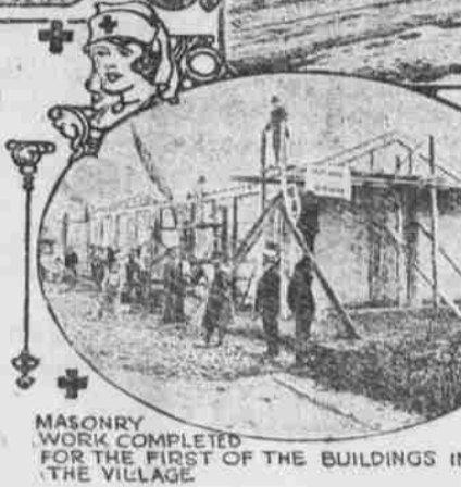
MASONRY WORK COMPLETED FOR THE FIRST OF THE BUILDINGS IN THE VILLAGE.
