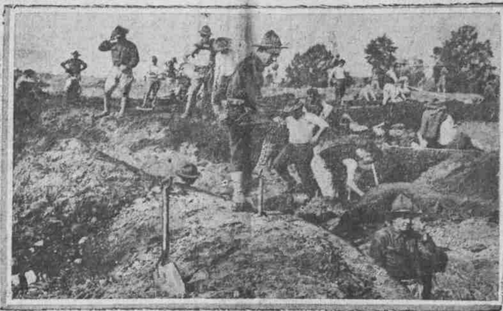
Guardsmen ready to do their bit for Uncle Sam, getting a touch of life on the modern battlefield, digging trenches at Camp Wadsworth, Spartanburg, N. C.
