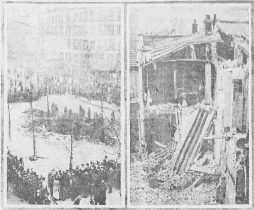
What a Bomb Did to the Subway. These photographs just received from Paris show the great damage done by the bombs thrown in the Zeppelin raid on Paris, Jan. 29. One bomb dropped on Rue de Belleville, dug a hole through the cement to the tracks. Another bomb tore a house apart leaving half standing.
