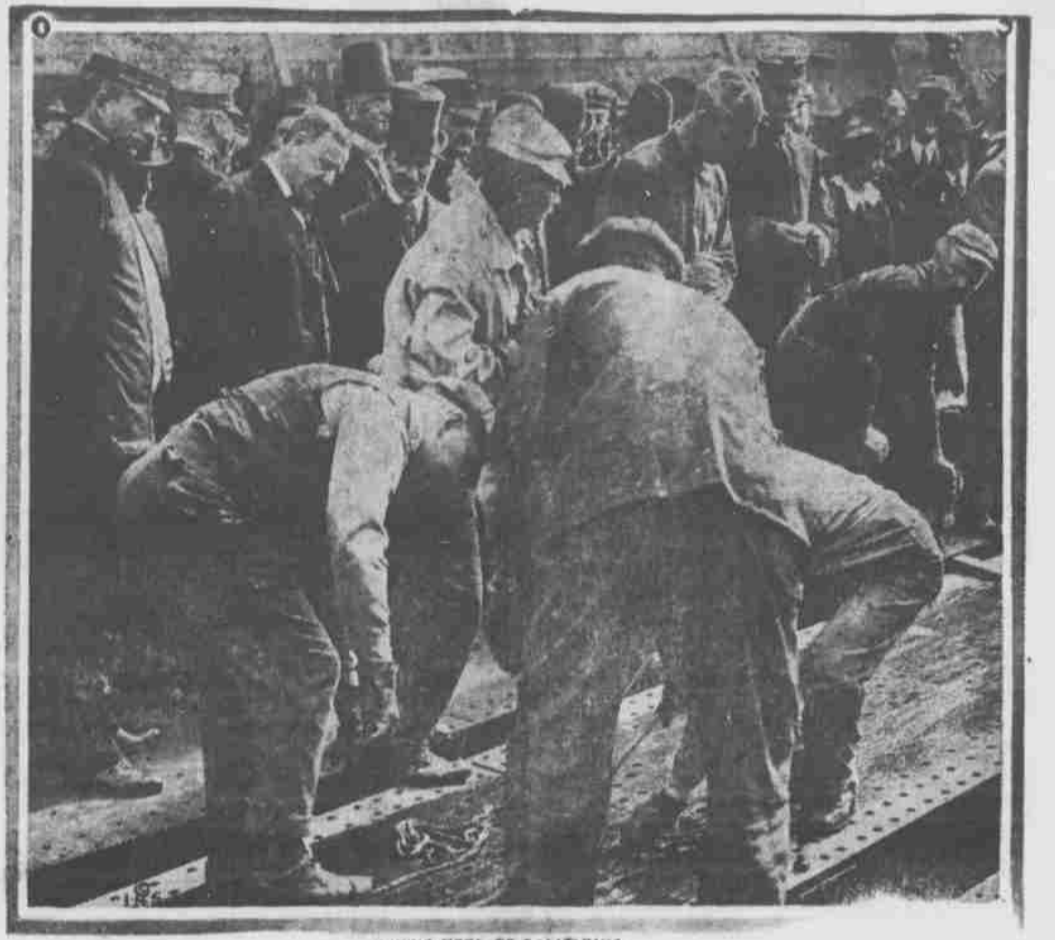
The picture shows Secretary of Navy Daniels watching the laying of the keel of the California, the largest fighting vessel in the world, at the Brooklyn navy yard. The California will cost $15,000,000 and will be run by electricity, furnished by dynamos driven by oil engines.
