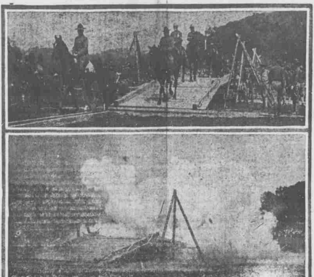
MAJOR GEN. O'RYAN AND STAFF CROSSING BRIDGE. BELOW
