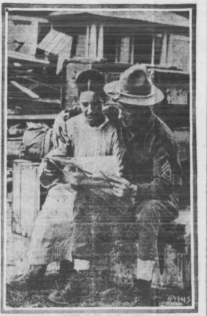
SERGEANT SHEPHERD AND WIFE. The picture shows Sergeant Shepherd, of the U. S. army station at Texas City, Tex., and his wife sitting beside the ruins of their home, which was almost completely demolished by the hurricane and flood which swept over the state, resulting in the loss of over 400 lives and a damage to property of about $5,000,000.
