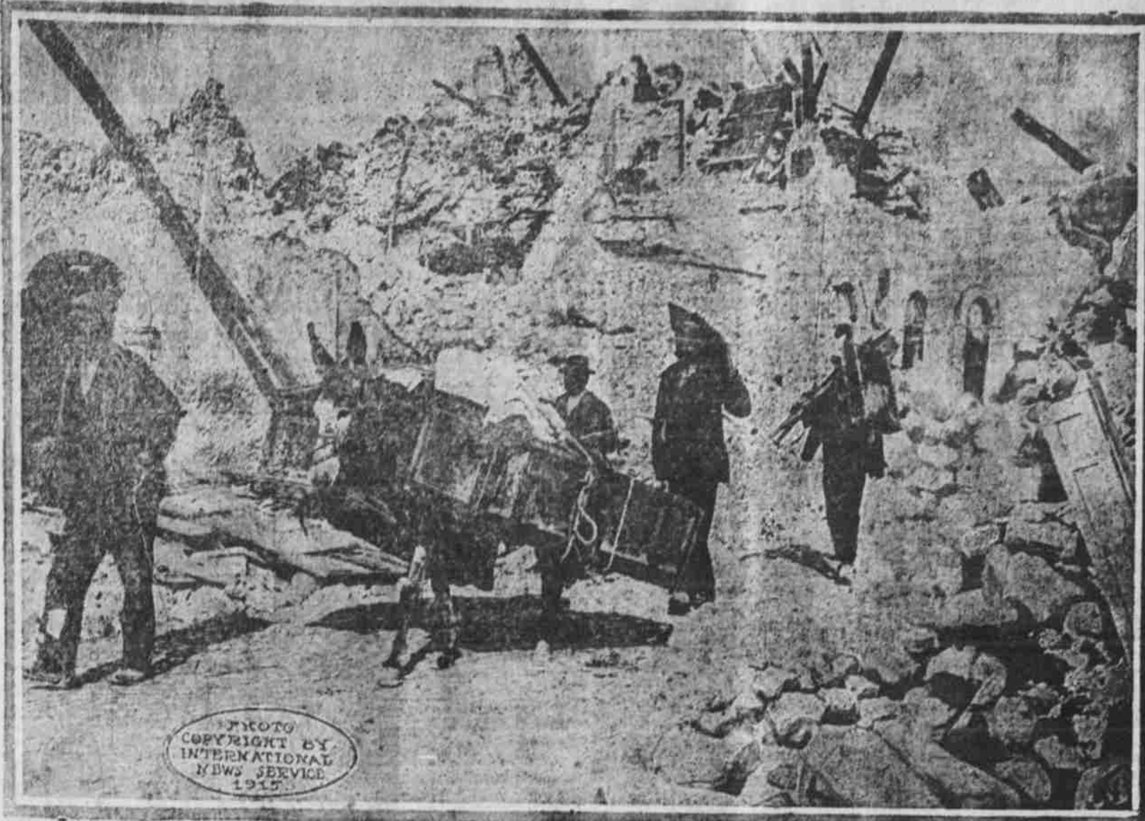
Photograph made the day after the terrible earthquake that wrought such havoc among the population and to the property of Avezzano, Italy. This photograph gives an idea of how the soldiers and the volunteer civilian relief workers went about the task of recovering the dead and wounded from the ruins and of preparing to rebuild their razed homes.
