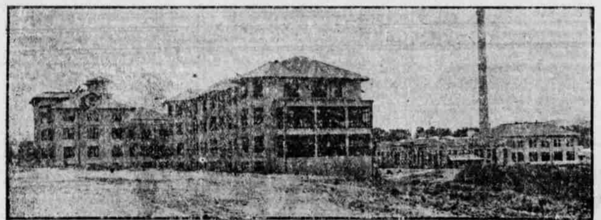
Side View Showing Laundry Building
