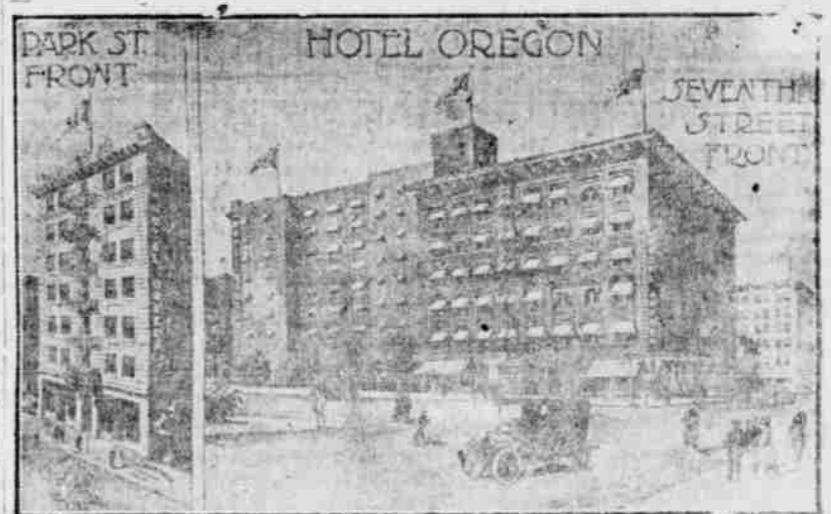
Located on the corner of Seventh and Stark streets, extending through the block to Park street, Portland, Oregon. Our new Park Street Annex is the only fireproof hotel building in Oregon.
