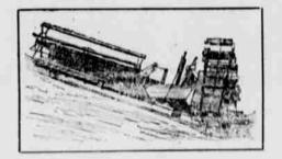
The cut above shows the side-hill harvester on a side hill. Note how it is able to stick to the side of the hill, while the header will slip down the hill. The main wheels are vertical, which braces the machine to the side hills. It works equally adapted to level land. The Holt harvesters are so'd exclusively in this section by
