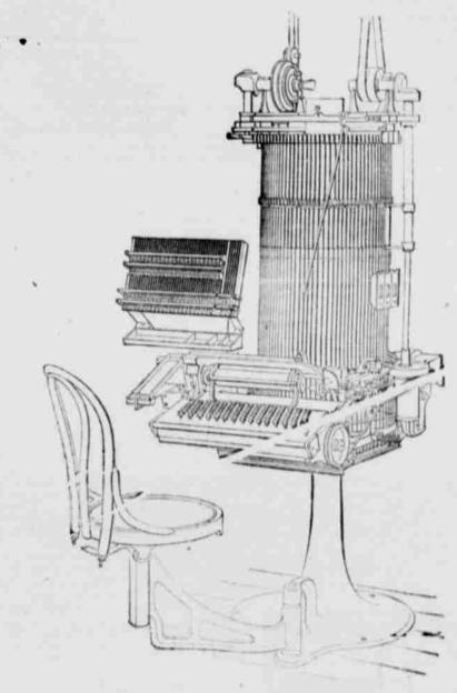
Machine is in good condition, requires only one quarter horse power to run it and with it one person can set from 20,000 to 25,000 ems brevier in eight hours.
