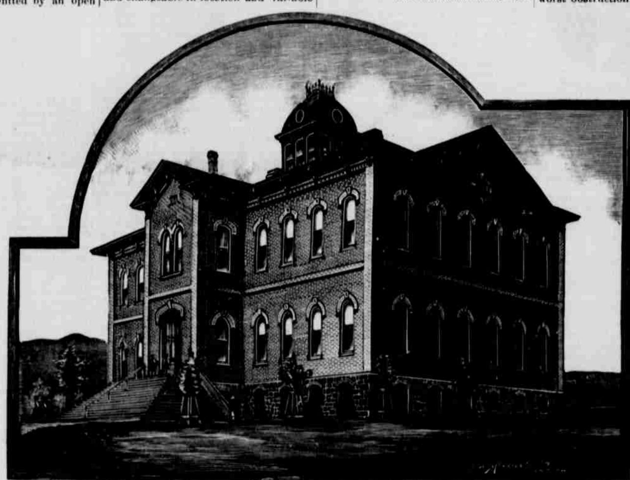
PUBLIC SCHOOL BUILDING AT PENDLETON.
