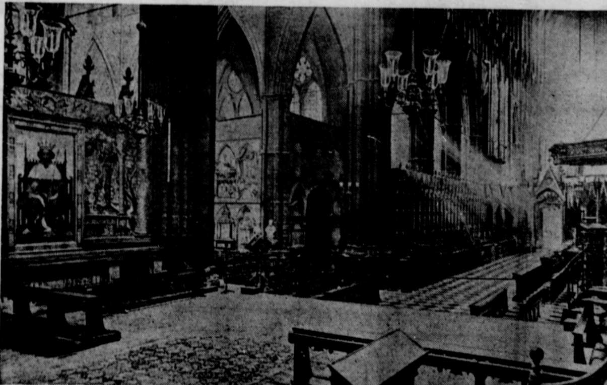
Reopened to the public recently, for the first time since the coronation of King George VI and Queen Elizabeth, Westminster abbey showed the results of some renovating and restoration work. For the first time in centuries, parts of the abbey were cleaned and portions of it restored. View shows the choir and the crossing. Many of the stained glass windows have been freed of the heavy coating of dust which had obscured them for generations.
