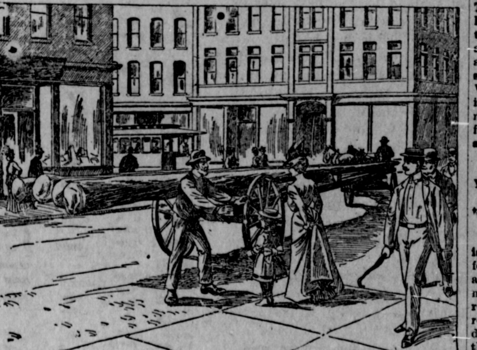
PILOTING LONG POLES THROUGH THE STREETS.
