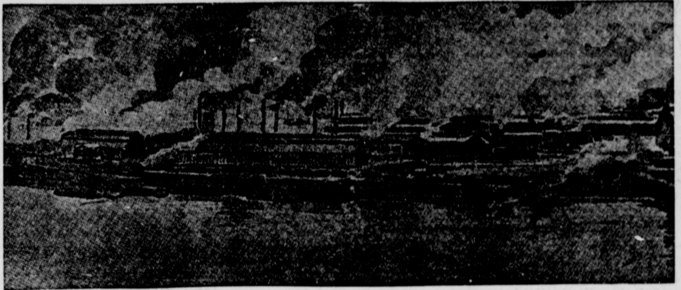
GREAT HOMESTEAD STEEL MILLS.
