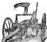
The greatest Labor-Saving Implements yet Invented. Vastly improved for Fall of 1877. 500 Sold in Oregon in One Year. EASTLY OPERATED. So constructed that by a slight motion of the Lever Plow made. EASILY OPERATED. So constructed that by a slight motion of the Lever the Plow is run out of the ground and raised clear, by horse-instead of man-power. It is stronger and less complicated than any other. Sole Agents for the well-known
