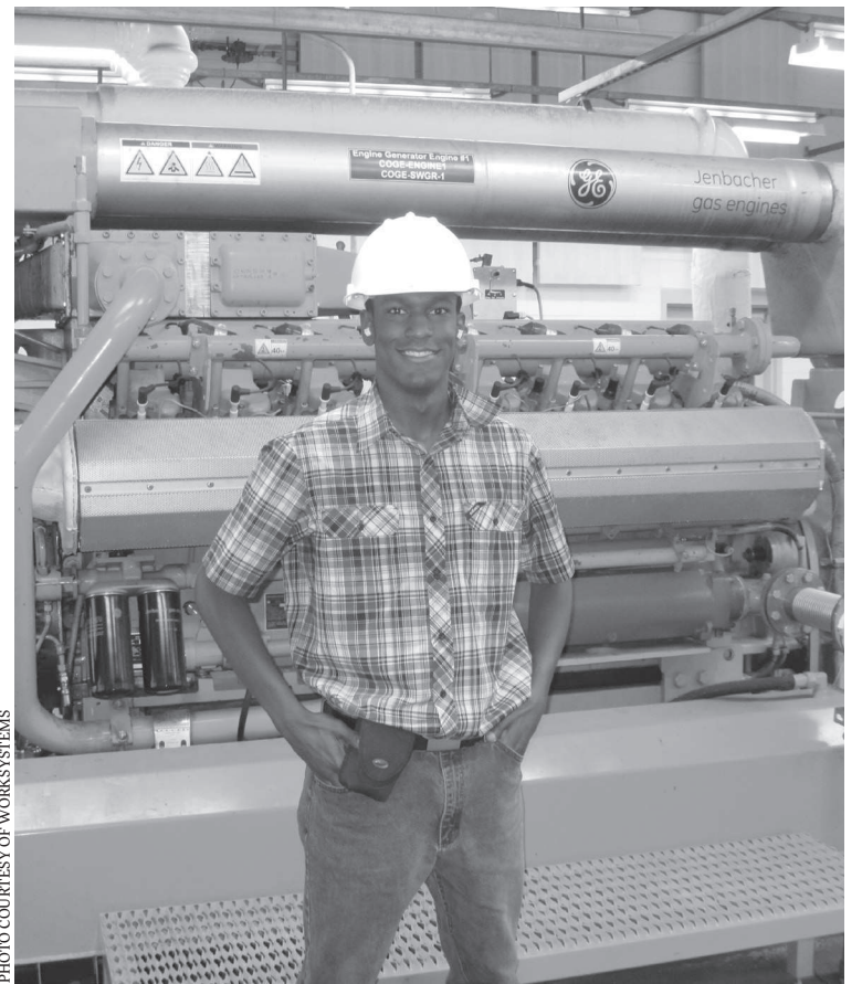
PHOTO COURTESY OF WORKSYSTEMS
