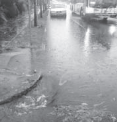
A storm drain on North Killingsworth overflows during record-breaking rain Tuesday afternoon.
