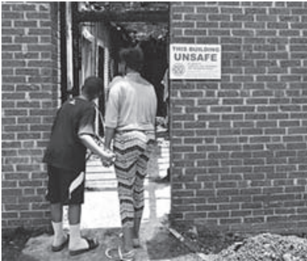
Elisha Walker, 9, and his mother Bonita Walker look at the charred remains of the back left wing of Briar Creek Road Baptist Church, June 24 in Charlotte, N.C. They are members of the church and Elisha had been attending summer camp since school ended for the summer. Investigators with the Charlotte Fire Department say a fire at the predominantly Black church is a case of arson.
