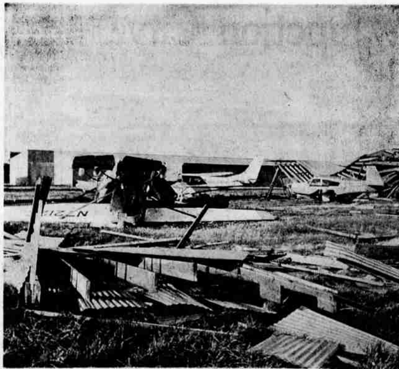
Seems that airplanes always try to fly away during a windstorm. This one did, but its moorings caused it to stay earthbound with heavy damage. Damaged hangar buildings show in the background of this scene at Mahlon Sweet Airport.
