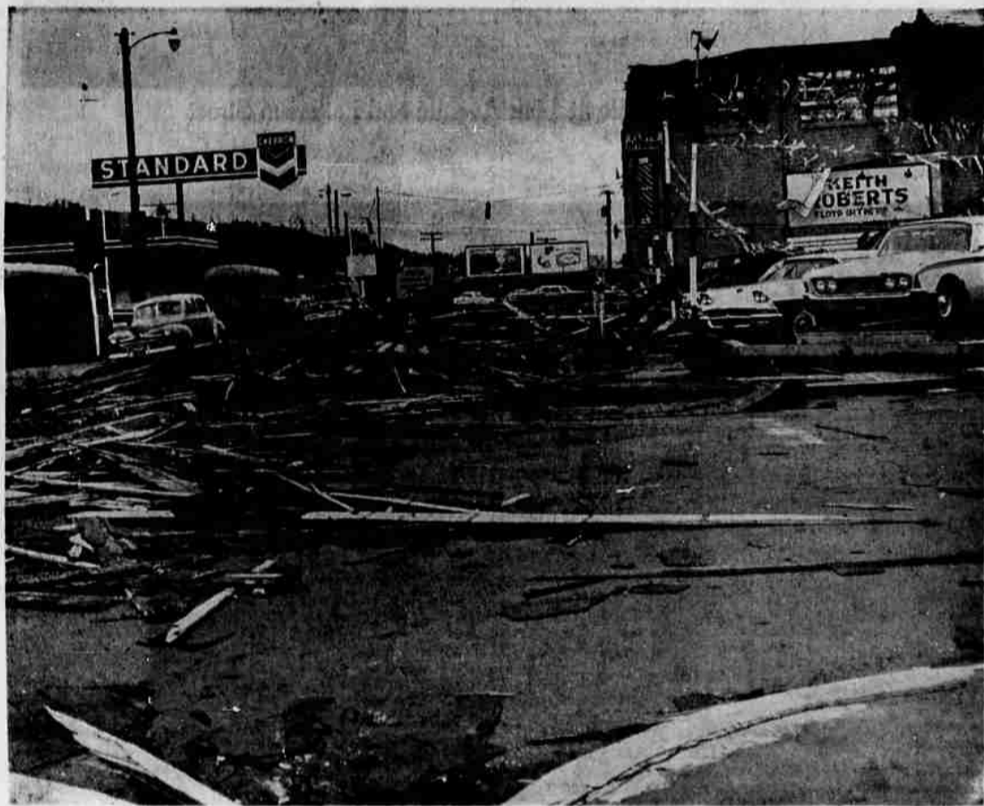
Debris litters street in front of Keith Roberts automobile showroom in Cottage Grove. Roof was swept off the two-story building by heavy winds Friday. Flying boards also damaged used cars in the lot next to the showroom.
