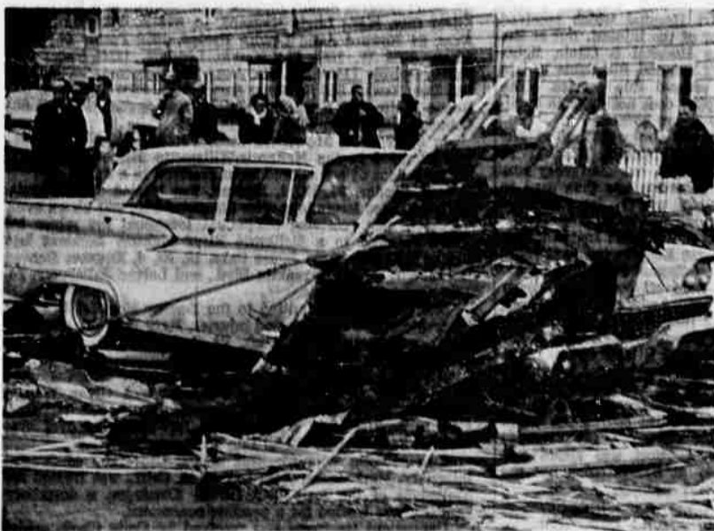
Another damage scene was at the Amazon housing project for married University of Oregon students. One student was killed by flying debris from the roof of nearby Roosevelt Junior High School. This car was stopped cold by flying lumber.
