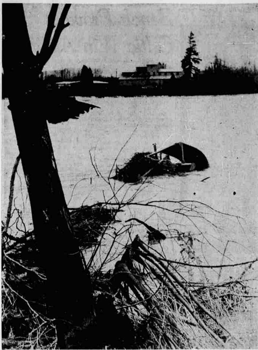
'CATS' DON'T LIKE WATER—The "cat" shown above, sticking partially out of the Willamette River, really got wet last weekend as torrential rains sent rivers over their banks. This bulldozer was being used at the construction site of the new Willamette River Bridge near Santa Clara. The "dozer" and a power shovel were completely submerged as the river level surged upward, but were becoming visible again Monday as the waters dropped.
