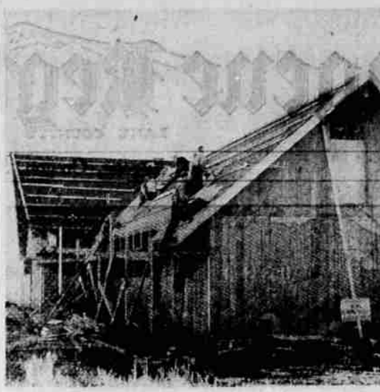
(Register-Guard photo, Willamette ev.) "GRAB A HAMMER"—The note that comes with this picture of the new building for Willamette Evangelical United Brethren Church, says: "We are really in earnest about building a church out here north of the Ferry Street Bridge. If you don't think so, put on some old clothes, grab a hammer, and come on out." The interior work is well under way, and moving-in has been set for April 3. Saturday, Tuesday, and Wednesday are work days, and the Ladies Missionary Group serves dinner to all workers.
