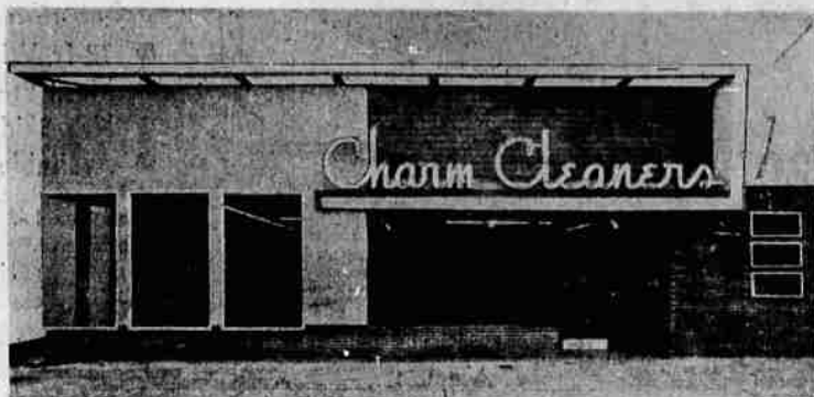
One of the most modern plants in the Northwest at 1469 Willamette — where there is always plenty of parking space right at the front door.
