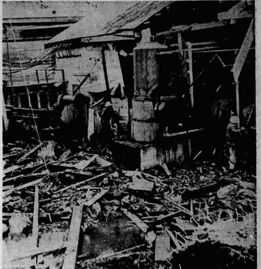
BLAST DAMAGE—The boiler room of the Co-op mill at Swisshome looked like this when smoke from an explosion cleared Wednesday. State Highway Department crews were blasting to straighten a dangerous curve ½-mile west of Swisshome when the charge went off. Debris blocked Highway 38, which was reopened to travel Friday, tore out power and communications lines and heavily damaged the mill. Mill officials declined to make a money estimate of the damage but said 170 persons would be out of work for a time. An official said it will take about a week to repair the mill and perhaps an additional week to set up new transformers and bring power to the mill.
