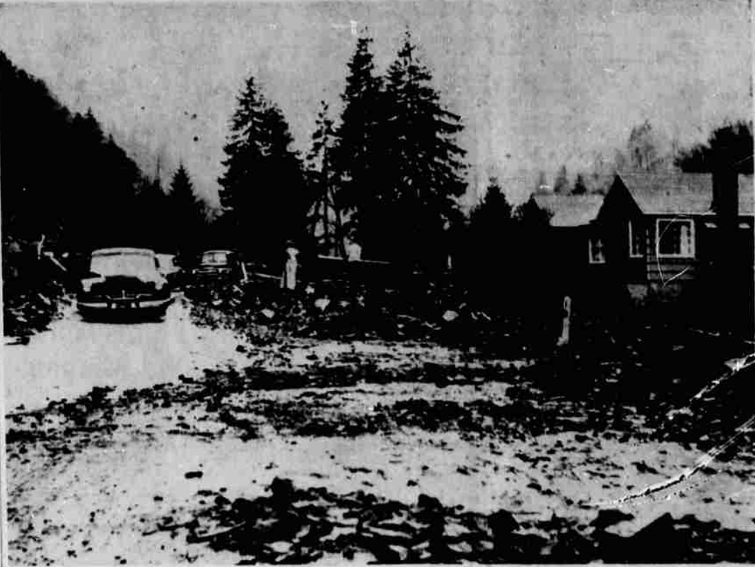
MAPLETON — The Ott Gossler place was surrounded by a sea of mud Friday morning after a slide nearly took the house on a trip into the Siuslaw River. The debris and dirt which slid down the mountain from Berkshire Creek barely missed the Gossler place and the
