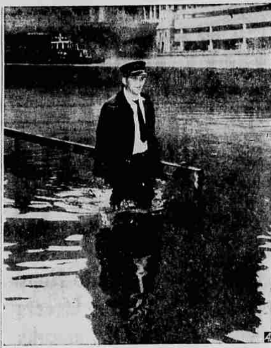
WORKING ON THE RAILROAD —You wouldn't know it, but fire battalion chief William Dinicola is walking on the Milwaukee Railroad tracks which lead into Chicago's Union Station. In background beyond retaining wall is Chicago River. The chief directed crews which worked all day pumping water from Union Station where partial service has been restored.
