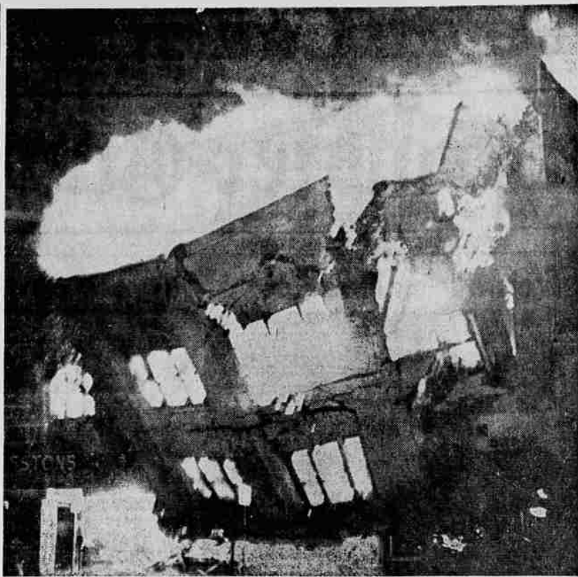
WALLS COME TUMBLING DOWN—The walls of the Milam Hotel and Livingstons drygoods store in Wichita Falls, Tex., are shown here as they crash into Indiana St. during a raging fire which wiped out three businesses and a hotel. Some estimates set the damage as high as a half-million dollars. His photo was taken by amateur photographer Perry T. Gresham.
