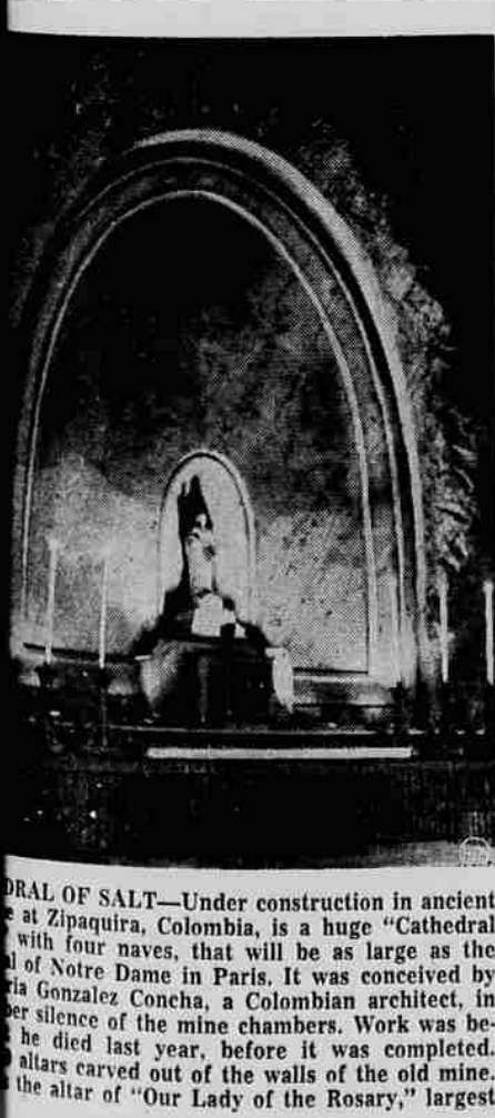
DRAL OF SALT—Under construction in ancient at Zipaquira, Colombia, is a huge "Cathedral of Salt" with four naves, that will be as large as the of Notre Dame in Paris. It was conceived by a Colombian architect, in the silence of the mine chambers. Work was begun last year, before it was completed. The altar of "Our Lady of the Rosary," largest
