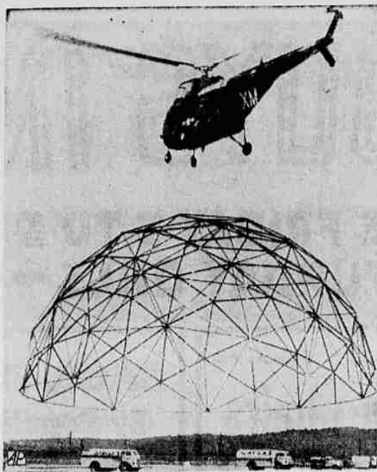
FLIES AWAY WITH ITS HANGAR—A Marine Corps HRS Sikorsky troop-carrying helicopter flies away a structure which had been its hangar a few minutes earlier, in a demonstration at the Quantico Marine Base.
