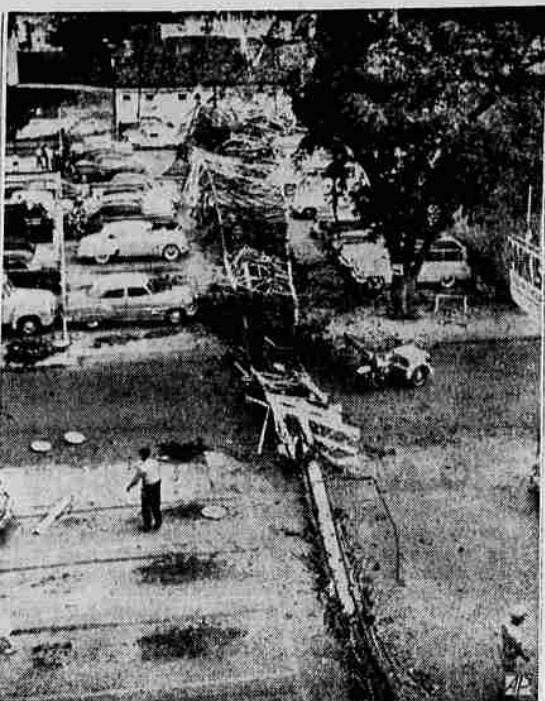
TWISTER FELS TV TOWER —A twister during a sudden windstorm in Mobile, Ala., hit a 435-foot tower behind the WALA-TV building in the downtown section and toppled it to the ground. It fell between two rows of cars in a parking lot—the only direction it could have fallen without crashing into a building. Several cars were damaged but no one was injured. The 85-foot television antenna on top of the 350-tower proper weighs 4½ tons. The tornado also tore off several roofs and blew out windows.
