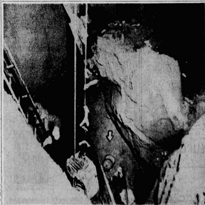
CAMERA CATCHES CAVE-IN—A huge mass of sand (at right) is shown falling on workmen in a sewer excavation in north Portland Friday afternoon. Wilburn Byers, whose cap can be seen at bottom center (arrow) was killed. Ted Suderburg, a rescuer, raises his arm to shield himself. Suderburg was saved by other diggers. The men were in the pit attempting to reach Pat Dennison, 35, the father of nine, who was killed in an earlier cave-in. The split-second picture was taken by Allen deLay of the Oregonian.
