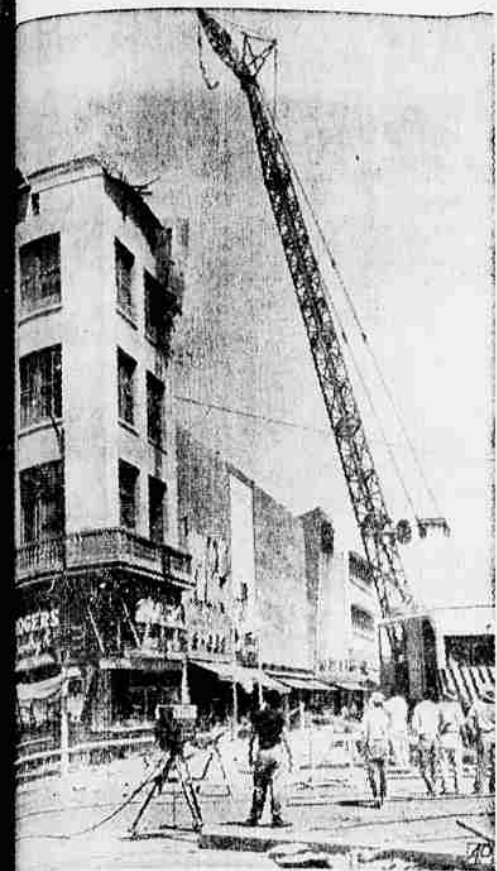
CONSTRUCTION WORK BEGINS — Workmen with huge cranes like this one began the work of tearing down unsafe buildings wrecked by the earthquake that shook San Francisco, Calif., killing two persons and doing millions of dollars in damage.
