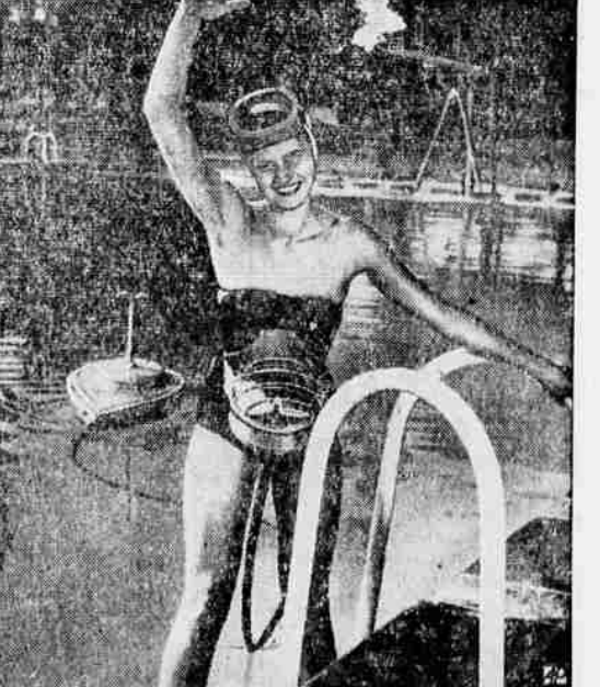
MOTORIZED SWIMMER —German girl in Munich wears a "water horse" propeller linked by cable to motor behind, and able to send her skimming along water at 10 miles an hour.
