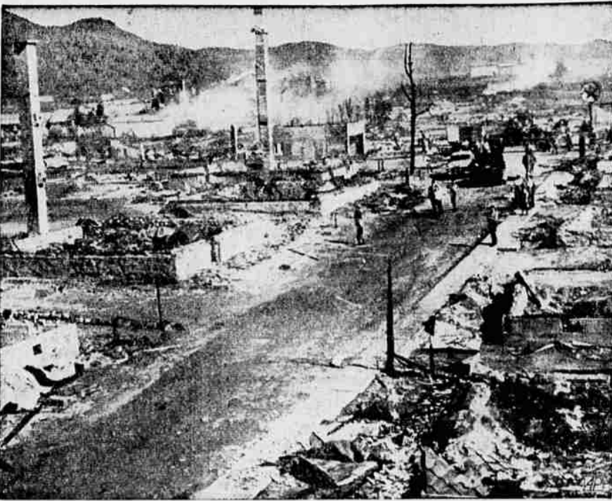
THE RUINS OF AT LEAST 52 homes and commercial buildings still smoulder after a fire raged through this rural Quebec village, St. Urbain. The fire started when a can of paint on a kitchen stove ignited in one of the homes. More than 350 persons were left homeless.
